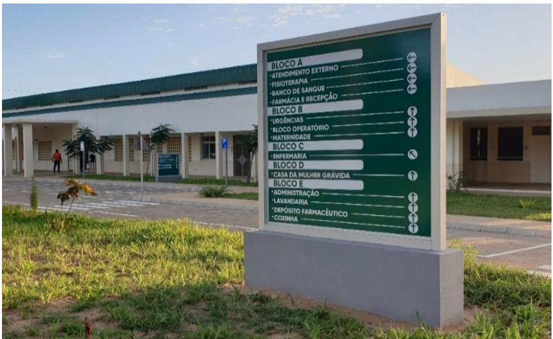
Hospital Distrital de Jangamo –Inhambane
